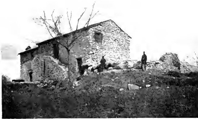
FIGURE 19. — THE HOUSE AND RUIN AT 58 From the southwest
